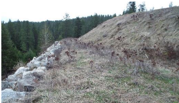
Lots 26, 27, & 28, Block #1, at the cul-de-sac end, are on a newer fill over an older slope protected by rip rap. (left)
